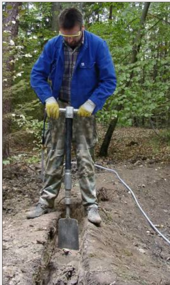
Digging in difficult clay - air-supply via utility vehicle
