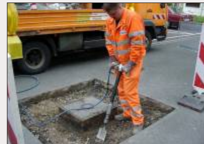
Removal of wet-mix macadam
