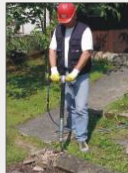
Demolishing concrete
