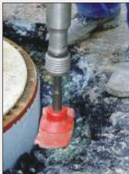
Compacting in narrow areas
