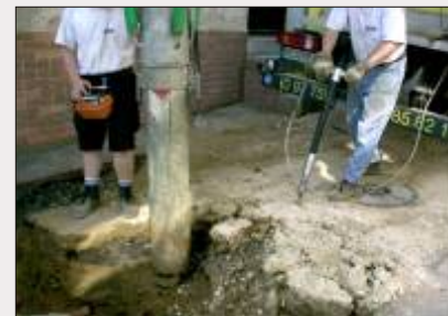
Loosening for suction excavator
