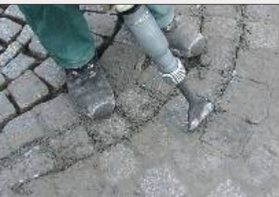
Cutting bounded plaster joints
