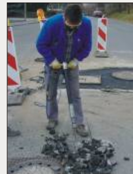
Breaking up asphalt
