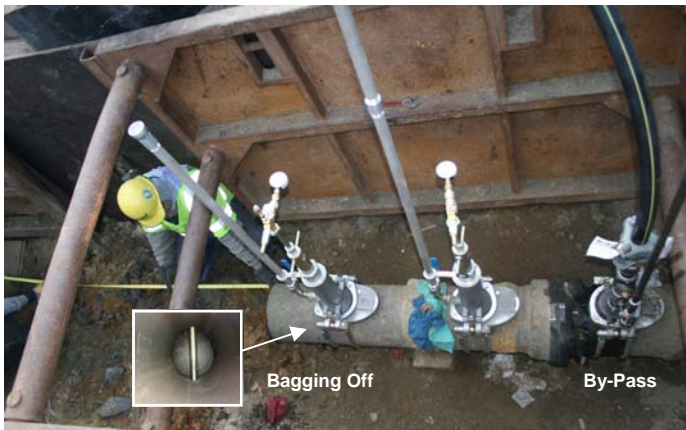
By-Pass Assembly and Bagging Off System for Gas Flow Stopping
