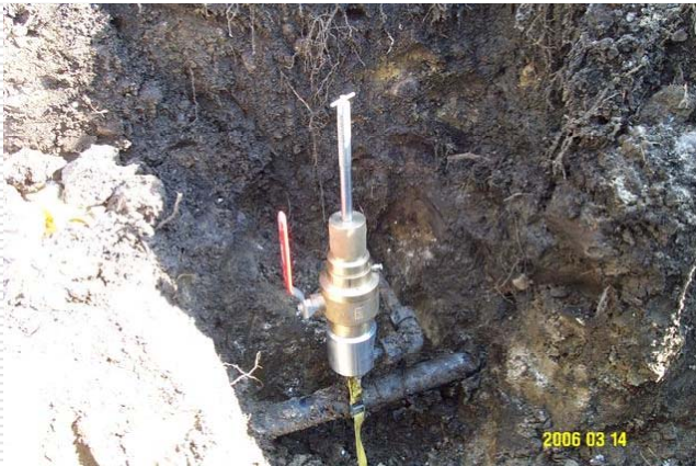
3. Cap is removed and an expansion stopper is installed into the throat of the tee.
