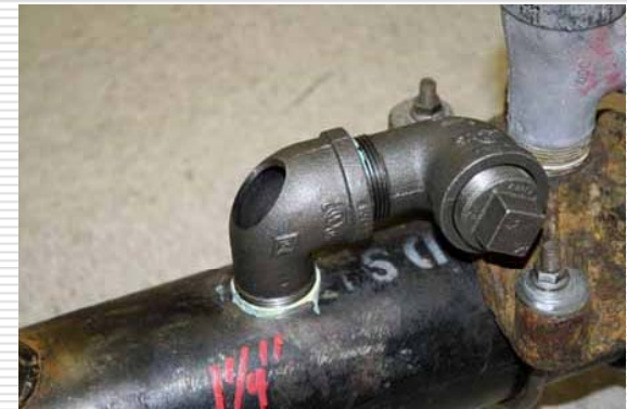
Swing joints, where the street elbow is threaded into the main.
