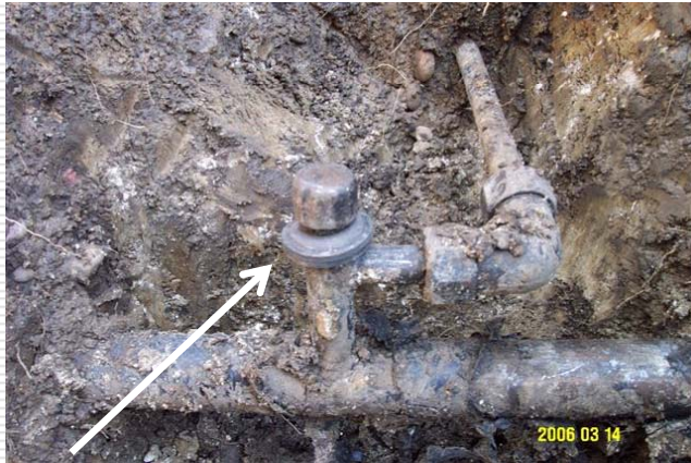
1. Beveled gaskets are fitted over tee cap.
