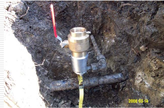
2. Half collars, housing, and ball valve installed.
