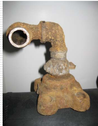
Tees that are attached to a corporation shut off
