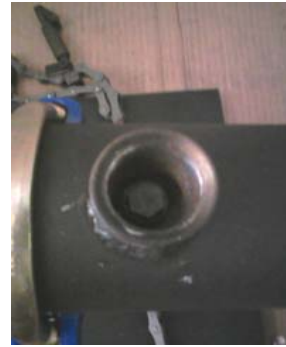
Once the inserted tapered threaded weld stops the flow of gas, assembly can be disassembled.
