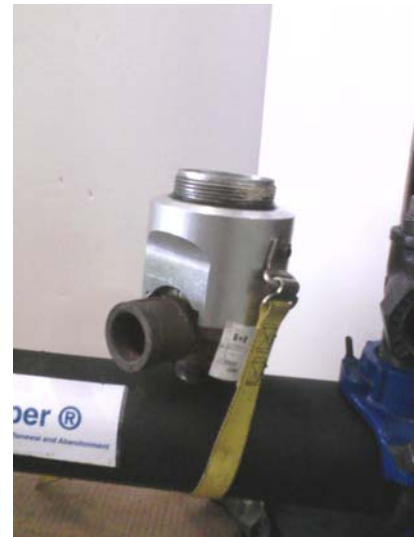
Fit cap housing over tee and secure safety strap.
