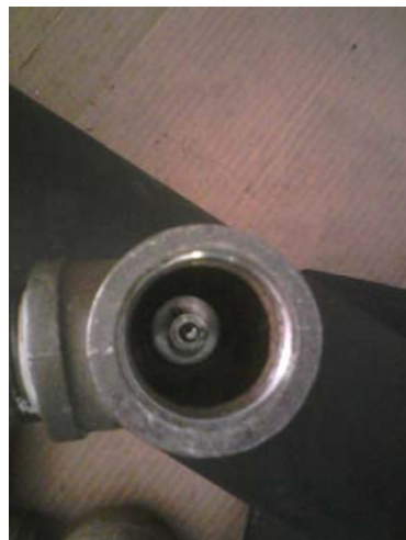
Replace malleable plug and disassemble entire assembly. Expansion plug shown in throat of tee for illustration purposes.
