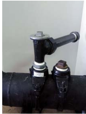
Place aluminum disc with embedded o-ring on top of the tee.
