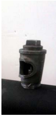
Before cutting off branch tighten plug and loosen tee. Plug should be tighter than tee. Cut branch.
