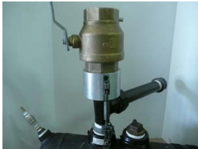
Street Tee threaded into a saddle.
