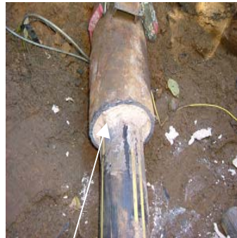
Cured Insertion Seal Foam after breaking out the main
