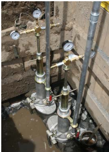
Simple Double Block and Bleed Operation
